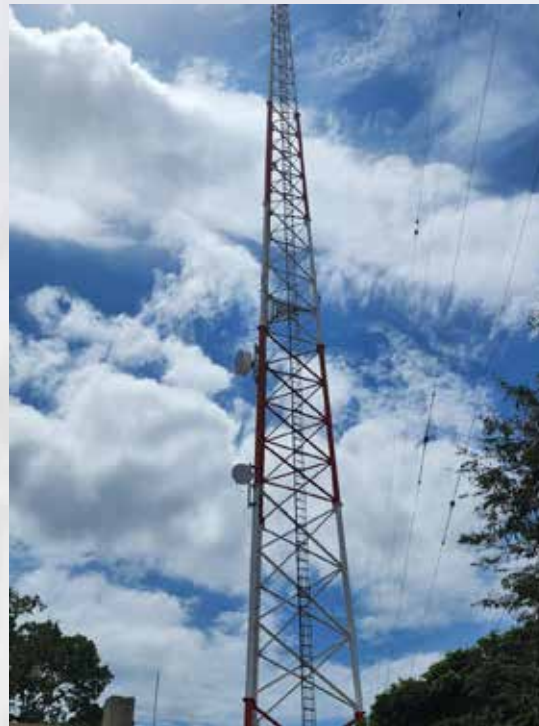
Figure 1 – The new self-supporting tower at Broadcasting House.
